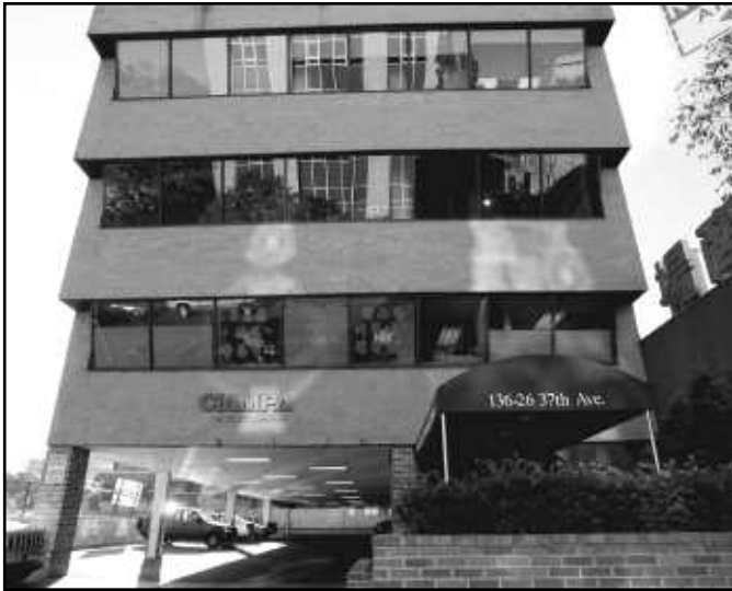
Ciampa Office Building
